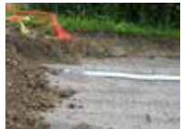
Gravel Base and Underdrain
