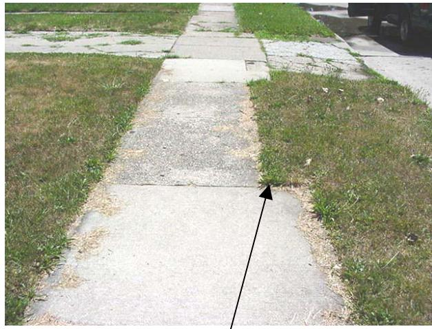
Variable width sidewalk – some areas still have 4' wide sidewalk. For the past forty years the standard has been 5'. All walk replaced during that time has been 5' wide creating trip hazards where the walk narrows.
