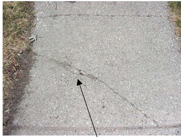
Cracked slabs – cracks in slabs, especially those with loose pieces of concrete.
