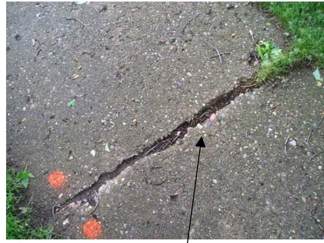
Spalled or deteriorated surfaces or joints – any area where the surface has pitted, popped out or spalled or where joints between slabs have chipped or deteriorated. These surfaces are hazardous and permit further deterioration from freeze/thaw cycles.
